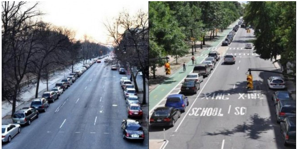
The insertion of a cycle track on this Brooklyn street dramatically improved safety for all road users without reducing daily car through-put. (Source: NYC DOT)
