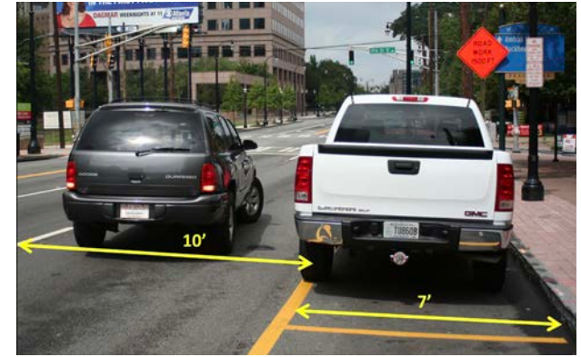
An SUV and a truck demonstrate that 10 foot lanes provide ample passing room, even against a narrow parking lane. (Source: Speck & Associates)
