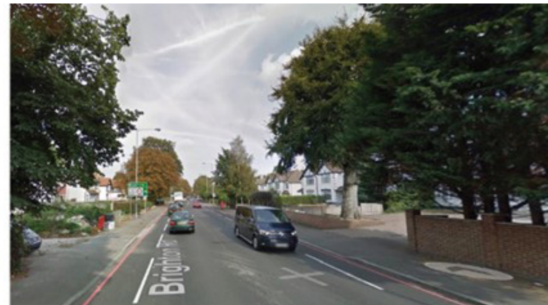
Removing centerlines from this and other British streets reduced driving speeds an average of 7 mph. (Source: Google Streetview)
