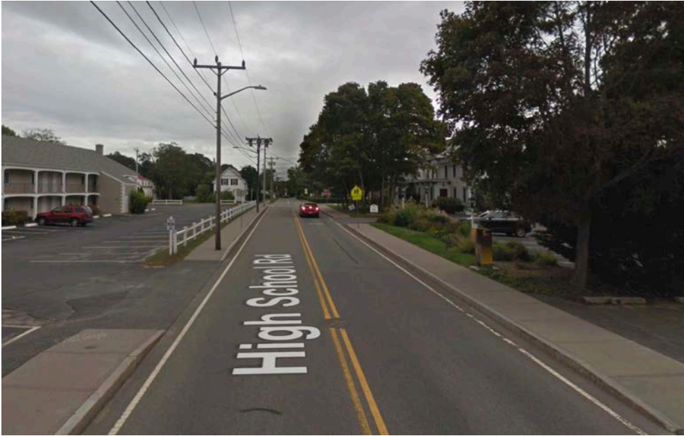
High School Road encourages high speeds with its highway-like geometry and is uncomfortable to people walking as well as biking. (Source: Google Streetview)
