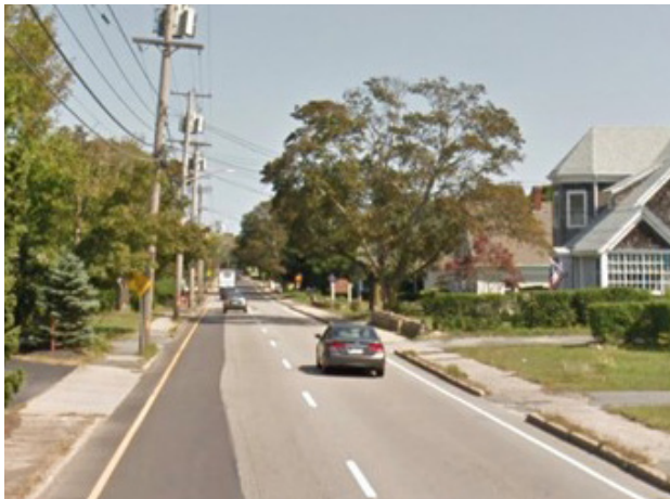
The absence of opposing traffic on South Street contributes to drivers’ propensity for speeding. (Source: Google Maps)
