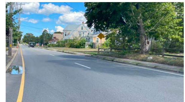
Lanes on North Street are 12 feet wide, a highway standard. Highway-style shoulders make them functionally even wider.
