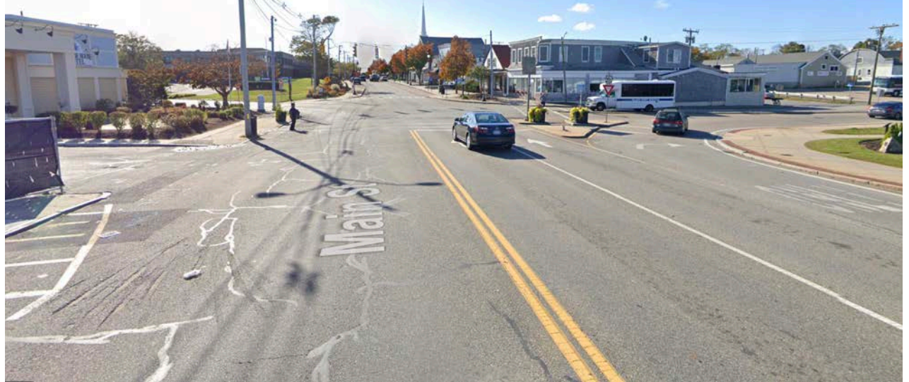
As it approaches Center Street in front of the Transit Center, Main Street holds 4 lanes in 67 feet of asphalt. Both the number and width of lanes can be reduced. (Source: Google Streetview)
